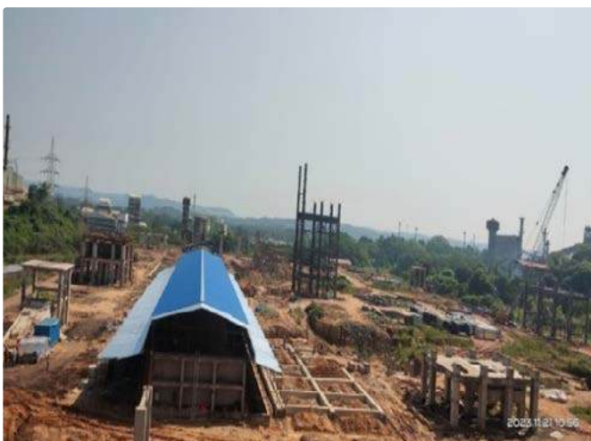
Coke Oven and DISP Projects
